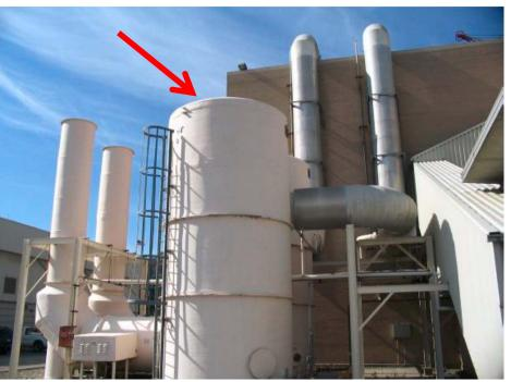
"The quad scrubber fans were running to provide ventilation of dewatering process areas, but the chemical feed and atomizing spray systems were not present nor in operation." Mill Creek Treatment Plant Odor Control Program Implementation, January 31, 2016
